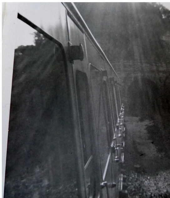
(emerging from Slade tunnel north portal)
