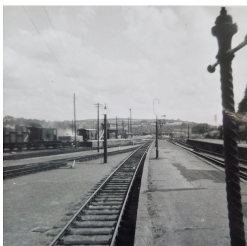
(Barnstaple Junction, looking towards Exeter)
