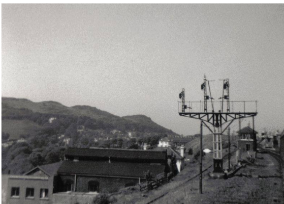
(the final approach past the dismantled signal gantry)
